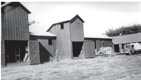
Ranch buildings at first Hamann farm Photo courtesy of John Turner & Richard Hermens
